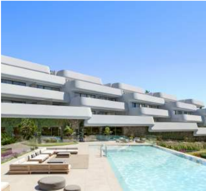
Large outdoor pool Amplia piscina exterior
